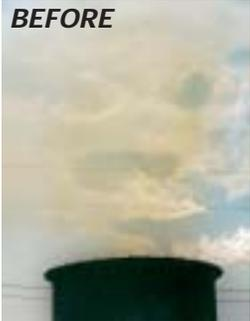
The top photo shows the emissions of a traditional high energy venturi scrubber. That same stack (photo below) displays no emissions after a MicroMist Scrubber upgrade.
