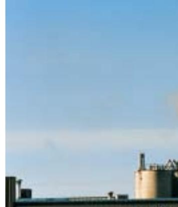
After adding micro-fine limestone conditioning tower, the secondary plume has disappeared. All that's left is the clear stack gas.
