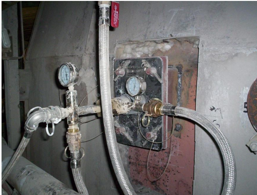
Figure 5. Lance Assembly With Lime Slurry Injection Port.
