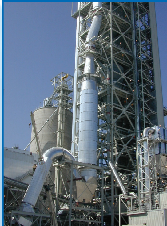
Gas Conditioning Tower
